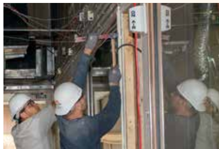
Workers in April begin renovation of space in Deputy Hall as the new home for mass communications.
