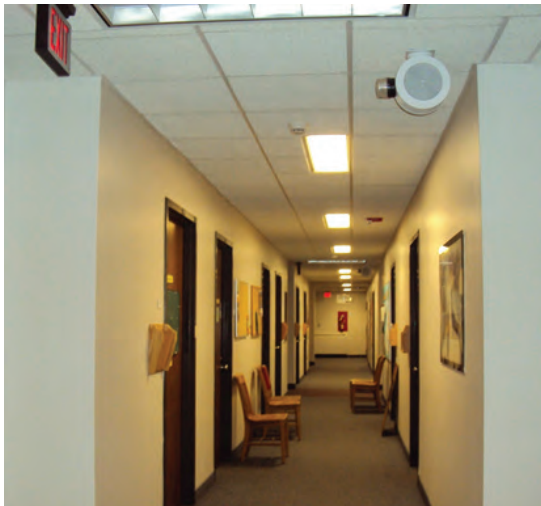
Current Hallway lighting
