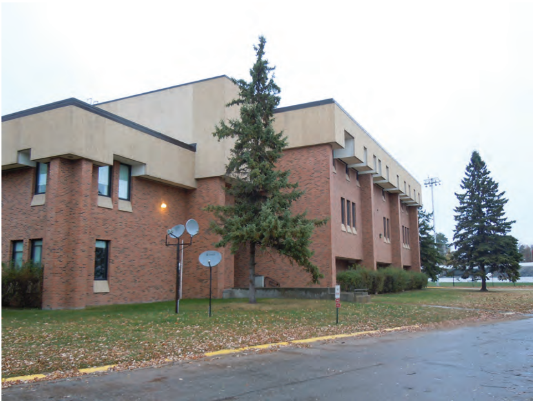
looking East from South side of building
