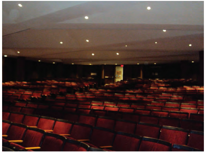
Lecture Hall lighting
