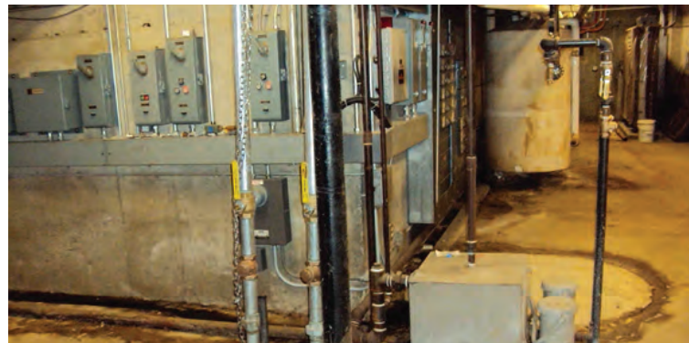
Current electrical gear and mechanical disconnects in basement
