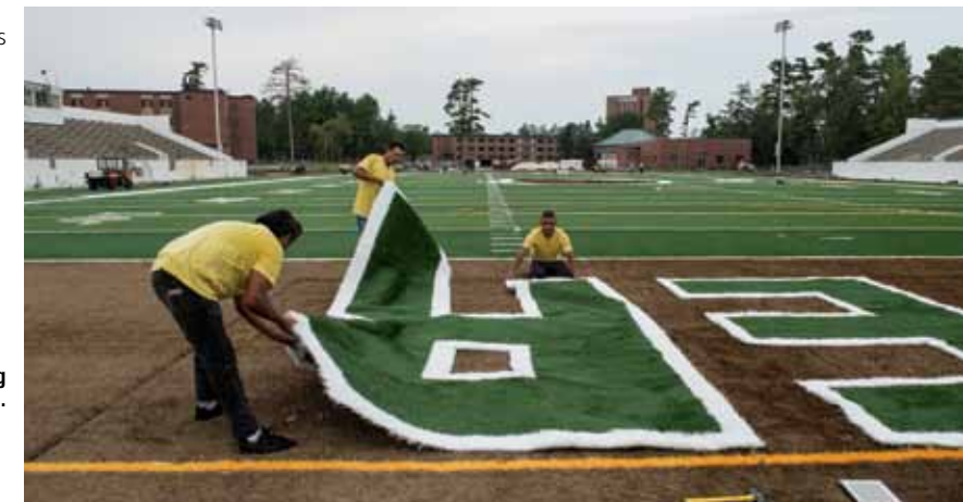
Workers install end zone lettering at Chet Anderson Stadium.
