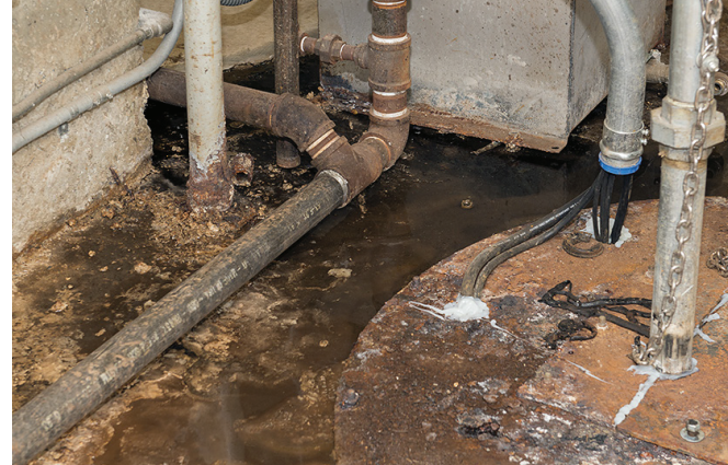
Water damage in the basement of the current Hagg-Sauer Hall.
