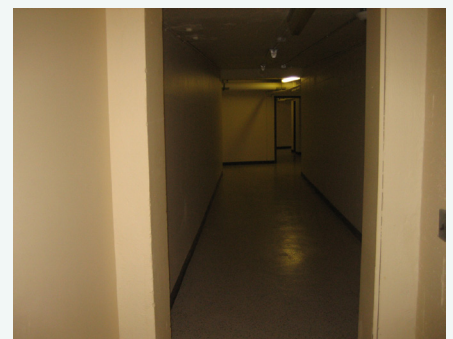
Tunnel Connection to Linden Hall
