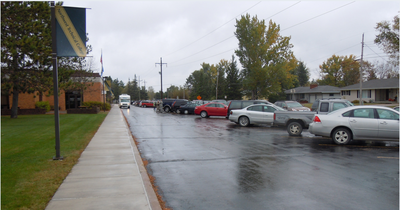
The main entry on the east side doubles as a parking lot, which undermines its sense of formal entrance.
