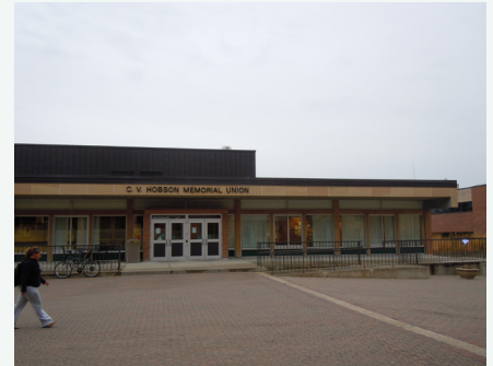
Exterior View (Lower)
