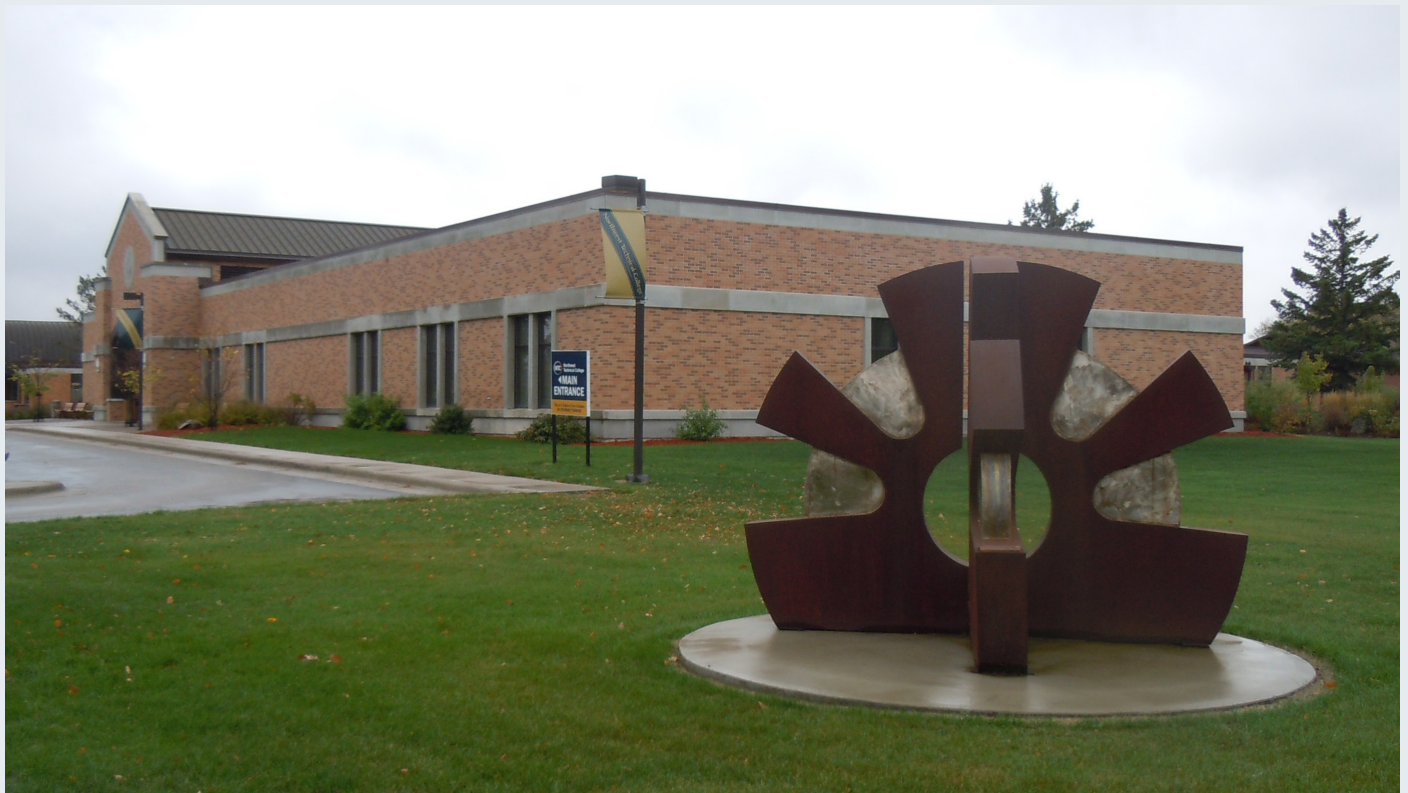
The Allied Health building and a large site sculpture help communicate the campus character.
