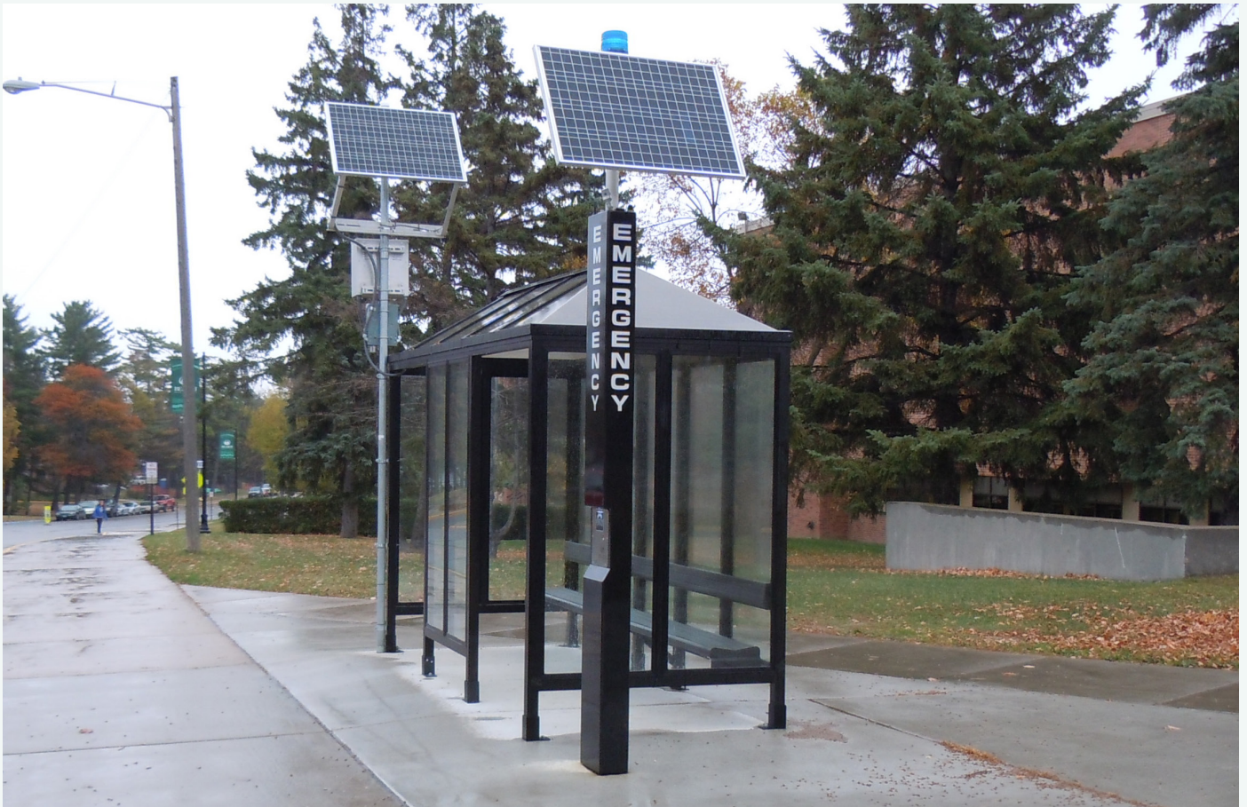
A bus shelter on Birchmont Avenue uses solar power for lighting and an emergency phone.
