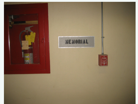
Signage at end of Tunnel
