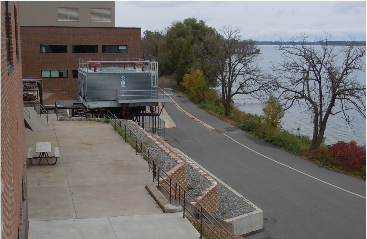
Service roads and other secondary uses occupy valuable lakefront land.
