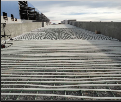
Figure 33: Integration of energy transfer pipe with piping under sidewalks and parking lots for snow melt.
