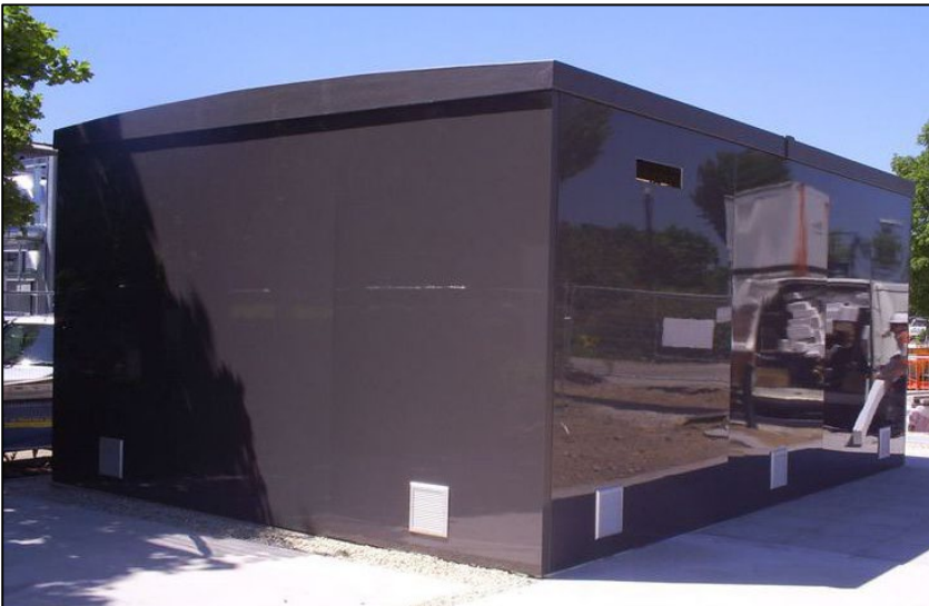
567 Figure 9: External modular mechanical room to house water to water heat pumps, and circulation pumps can possibly be located near the campus buildings.
