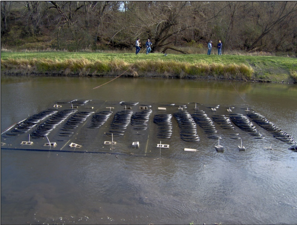
Figure 12: HDPE slinky surface water heat exchanger being sunk to the bottom of a pond.
