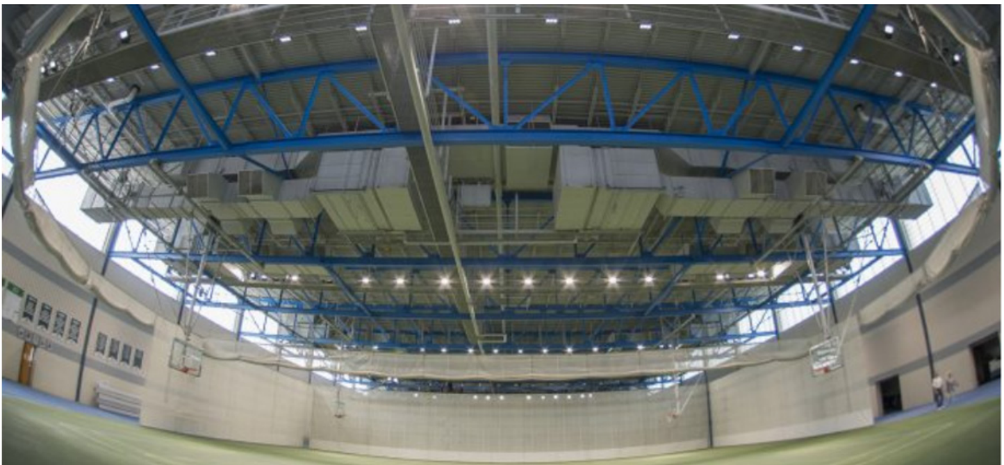
Through a partnership with Otter Tail Power Company, Bemidji State University is set to save thousands of kilowatt-hours of energy in the coming years, including projects like this lighting conversion as seen above.
