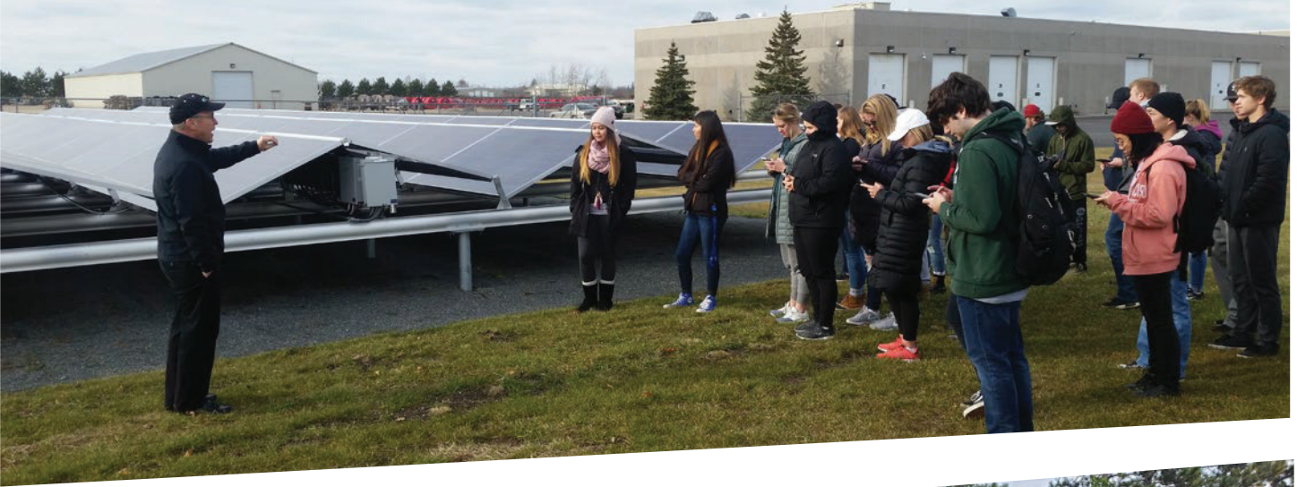
Sam Mason of Beltrami Electric Cooperative sharing with Bemidji State University students about the Northern Solar Community Solar Garden.
